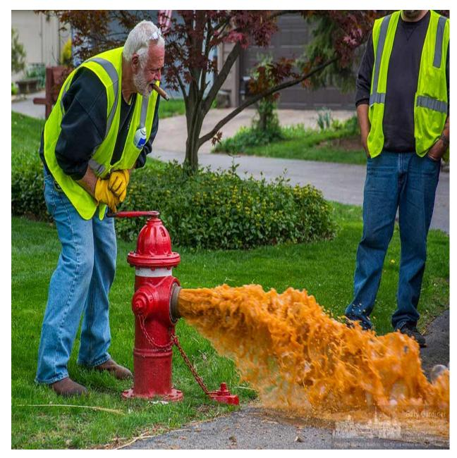
We will see coloured discharge which is normal. It can be black, brown, grey, rust or red. The crew will flush until water flows clear, readings reach a 5 NTU which should take 20 minutes per hydrant.
